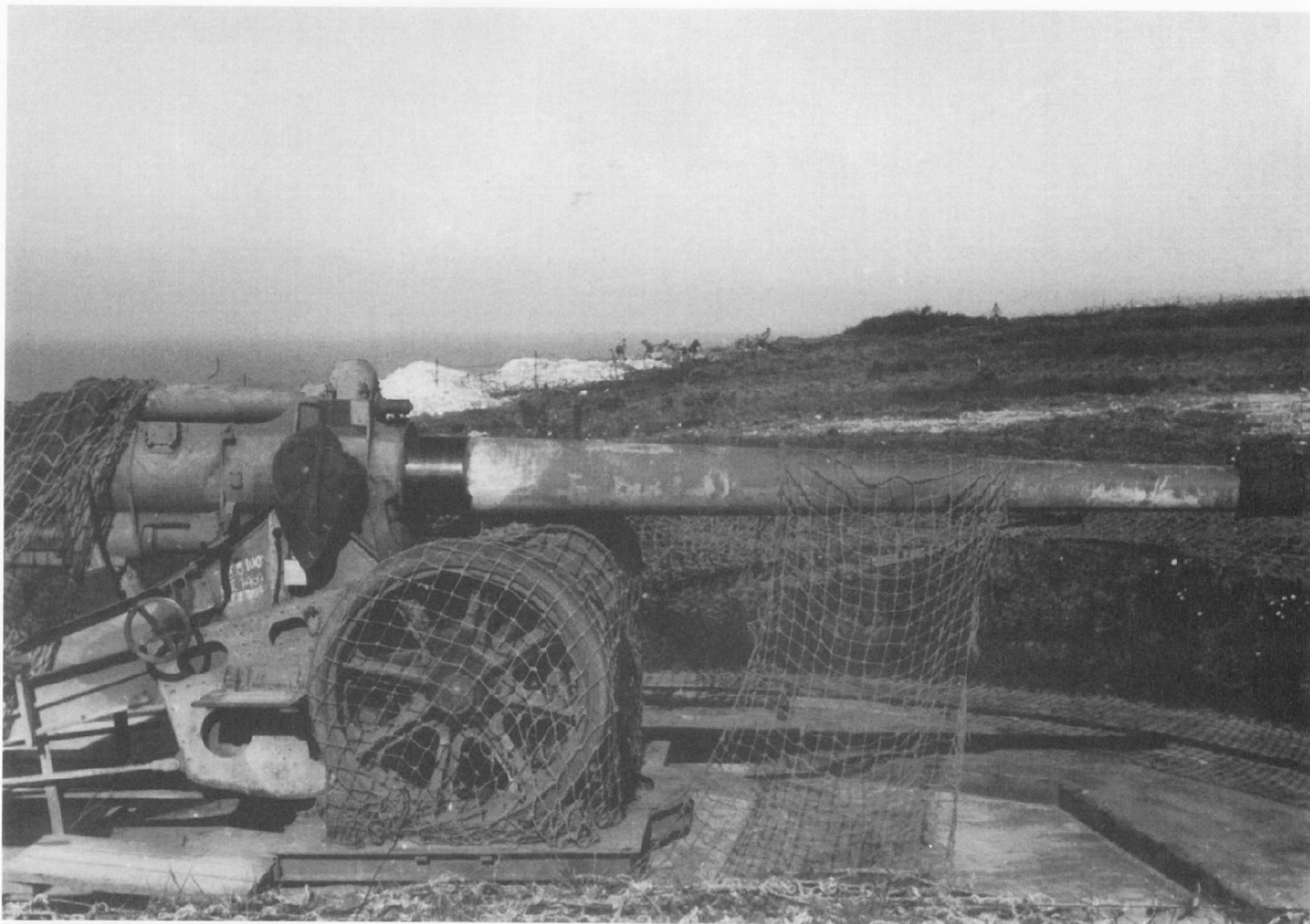
A 155mm Kanone 420 (f) of the Morsalines Battery in its ring mount. The photo was taken during construction in the summer of 1941. The concrete ring surrounding the base plate has yet to be built.
