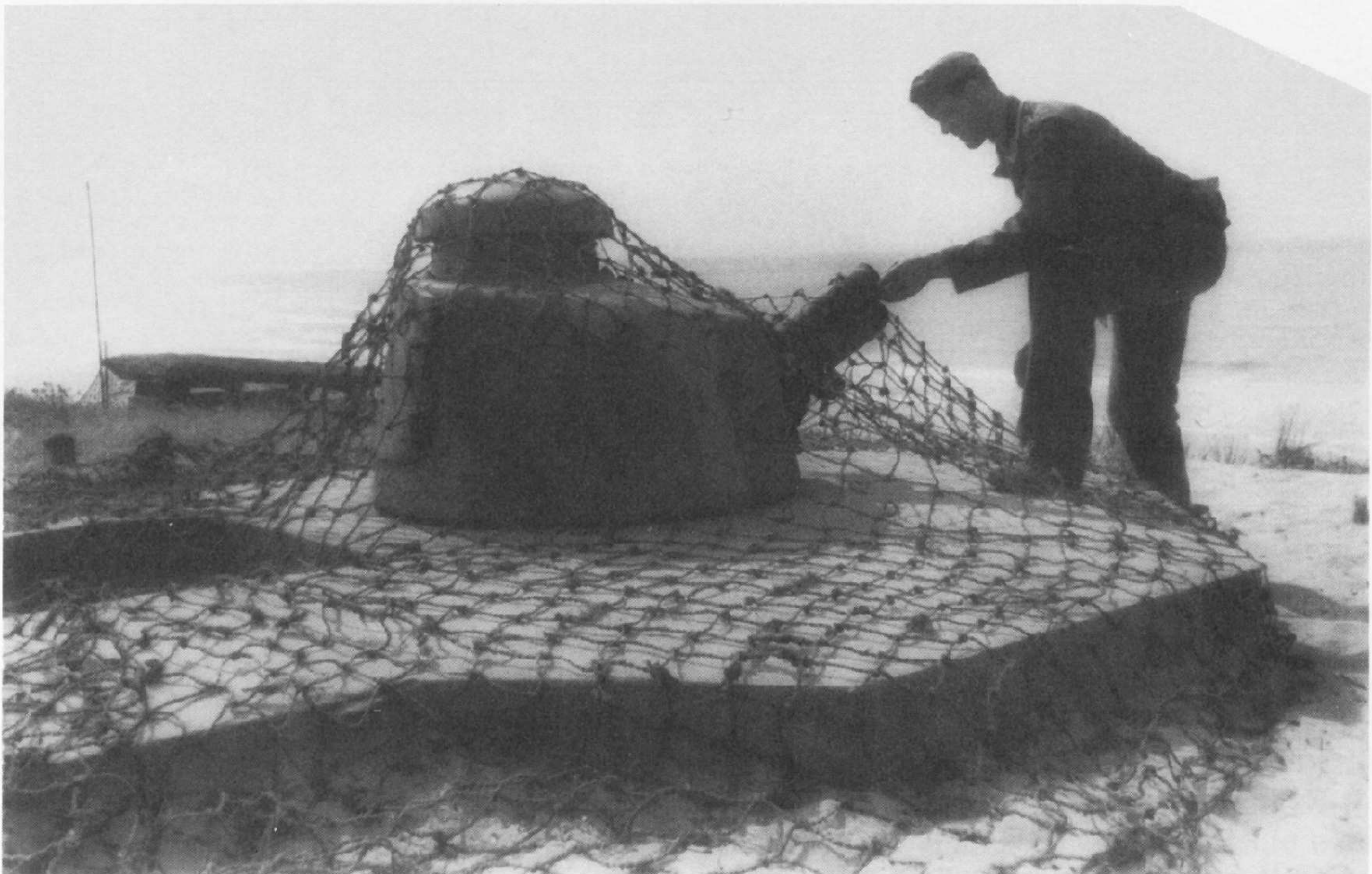
A Berliet armored turret with 37mm cannon on a ring mount in Resistance Nest 8 on the Cherbourg Peninsula.
