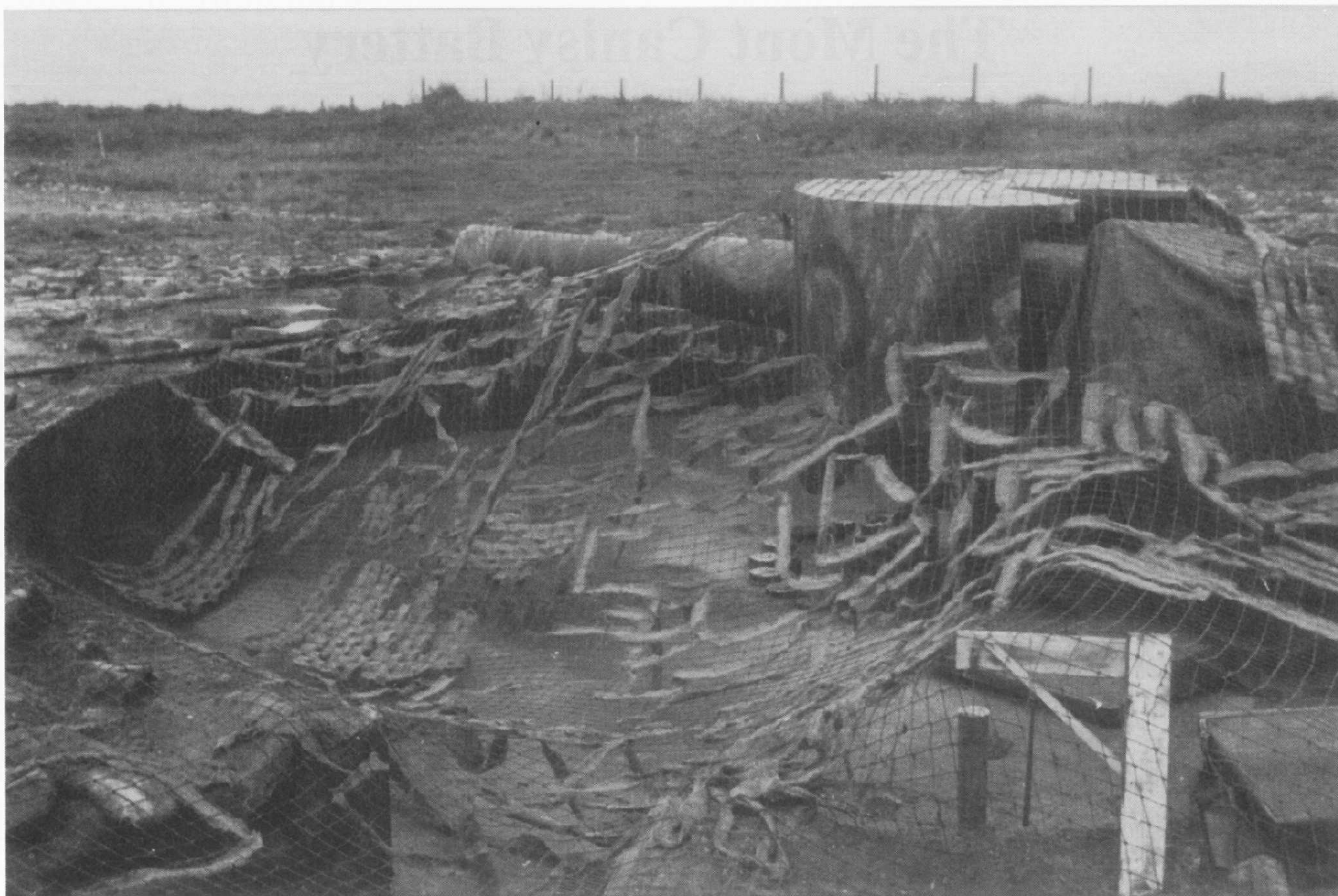
The 150mm SK L/45 was installed on the mount with its 100mm-thick armor shield. The gun received a camouflage finish of green-yellow in order to blend into the countryside. In this photo the muzzle and breech mechanism are covered with tarpaulins. (BA)
