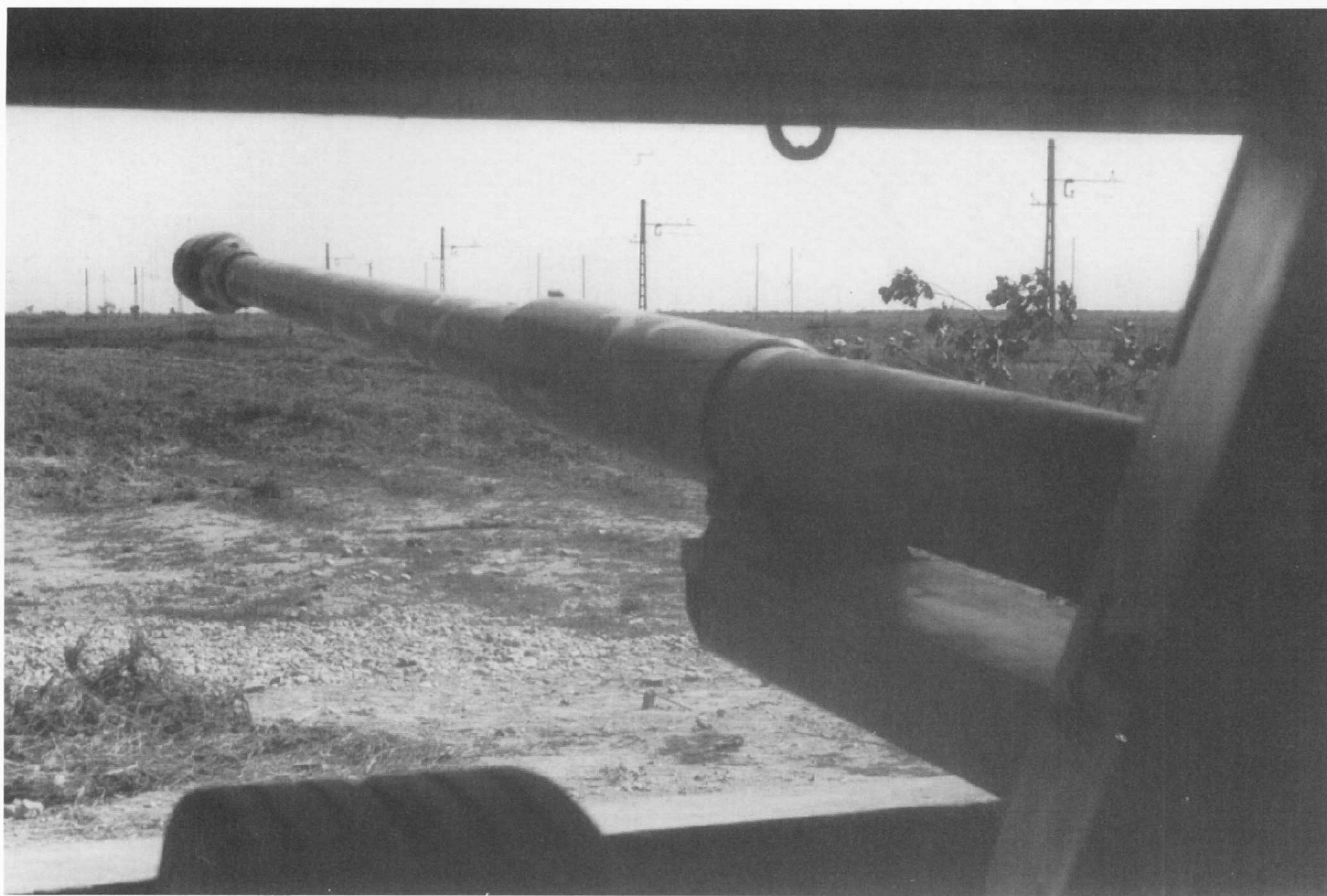
Only a small portion of the 6,616-millimeter-long barrel of the 88mm Pak 43/41 protruded from its bunker, which was placed in a flanking position, and even that part was screened by the flanking wall.
