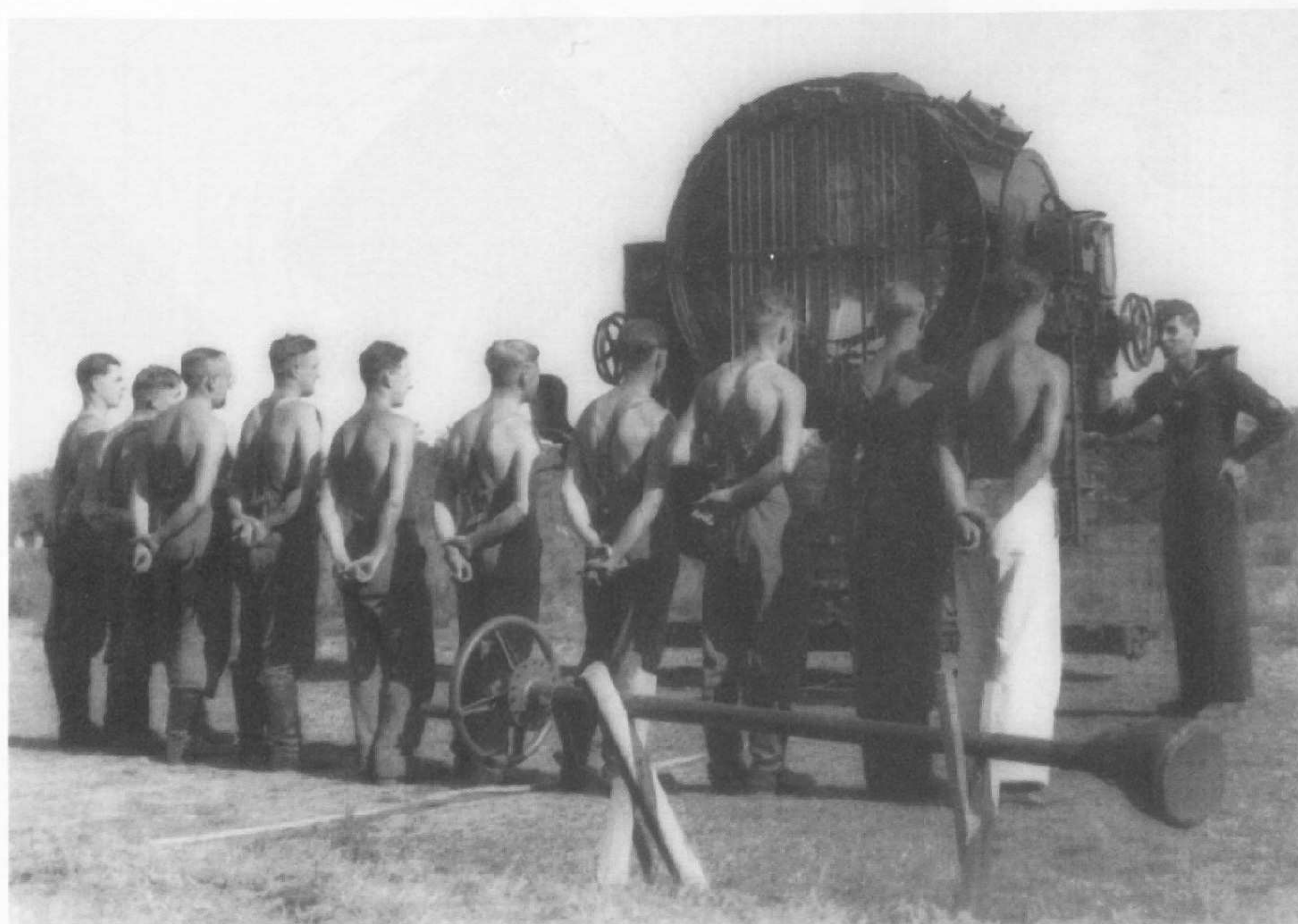
A 150mm searchlight belonging to the battery. In the foreground is the steering arm, with which one man could aim the searchlight in azimuth and elevation.
