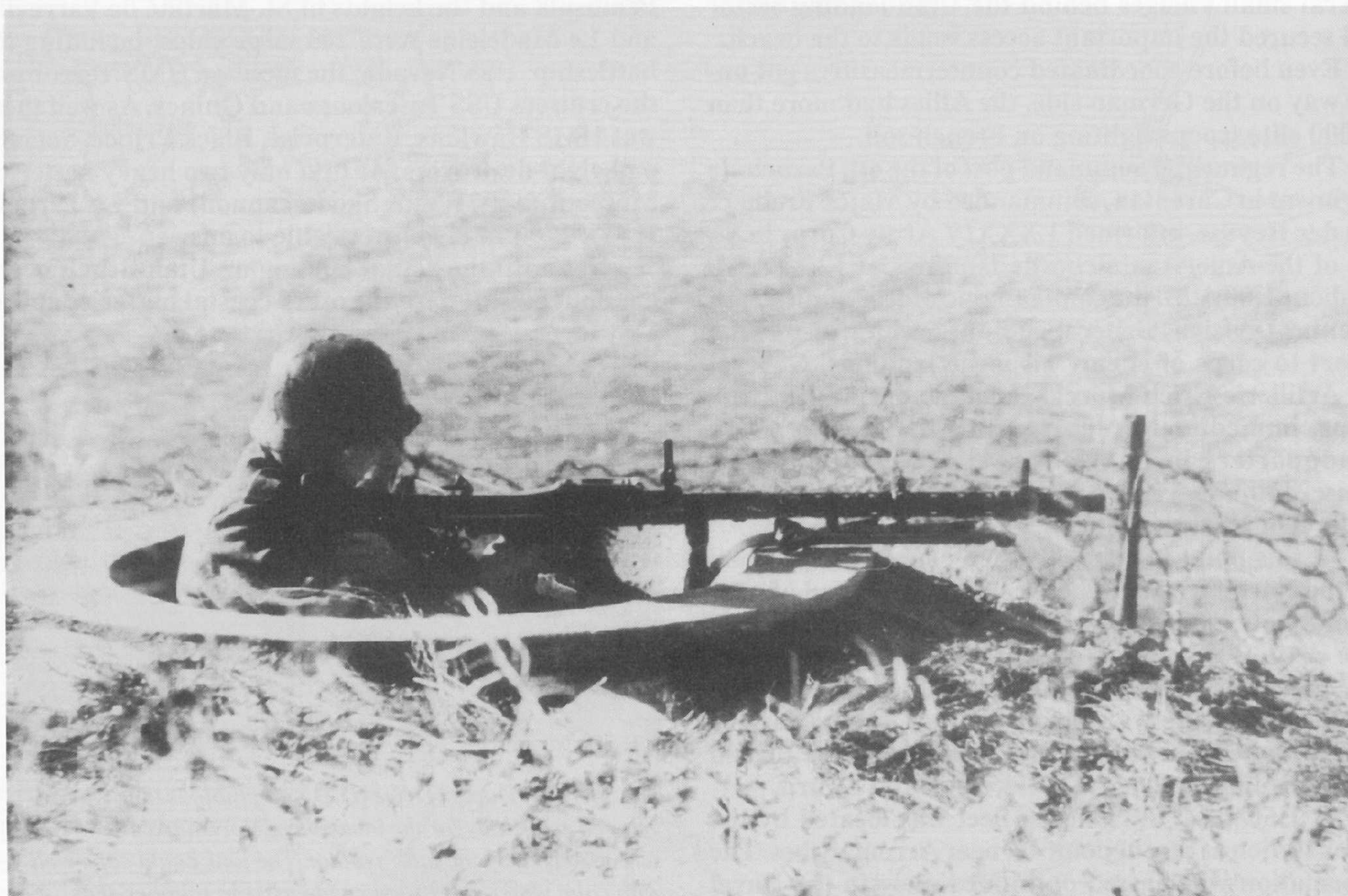
An MG 42 machine-gun in a ring position, Standard Structure 202, part of Resistance Nest 5. This tiny bunker proved extremely successful on account of its small size. 3.7 meters deep and 2.2 meters wide, it was very difficult to spot.
