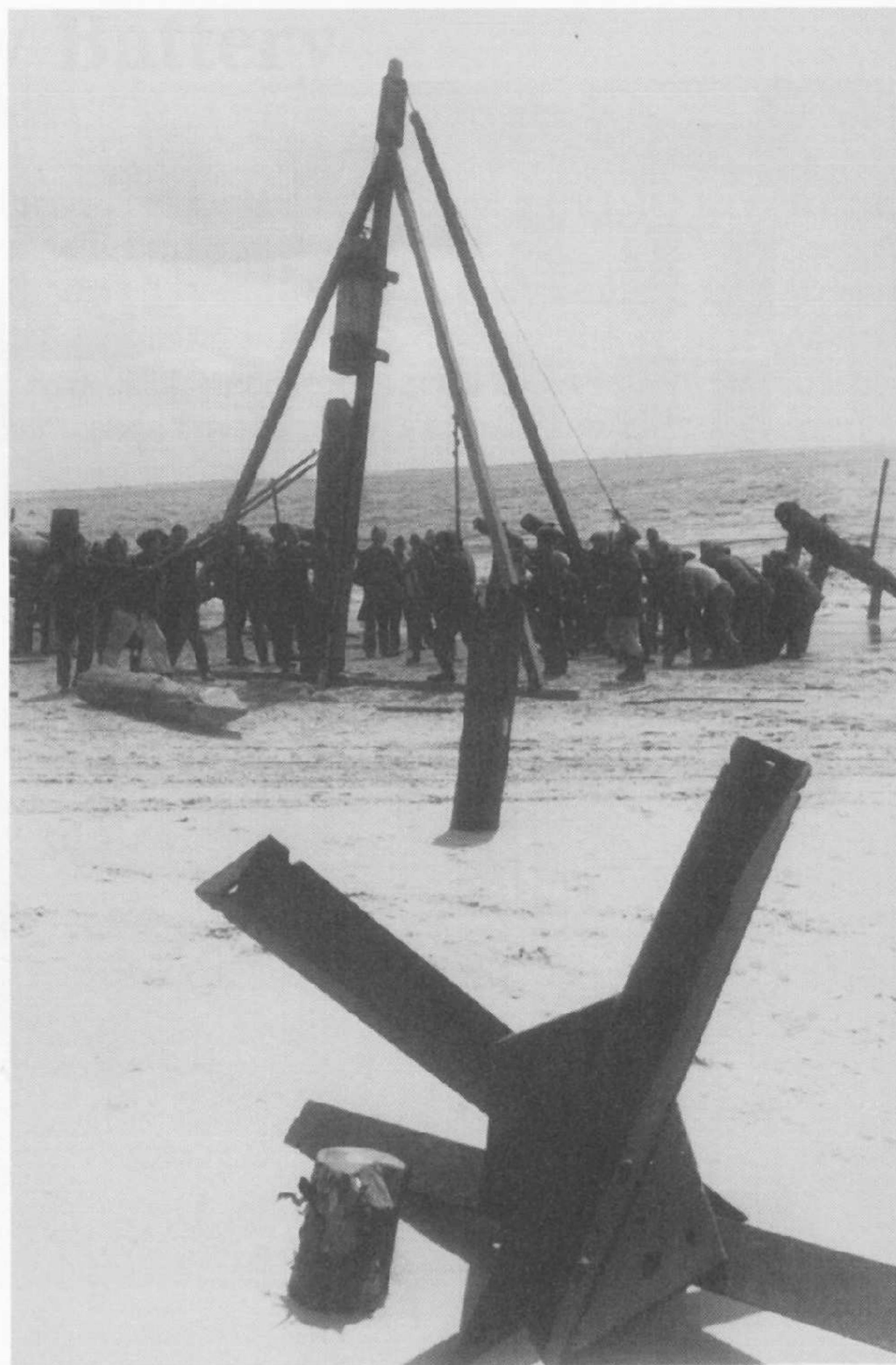
In early 1944 German combat engineers ram tree trunks into the outer beach near Lion-sur-Mer. Fitted with an anti-tank mine and steel blades, these obstacles were supposed to sink Allied landing craft.
