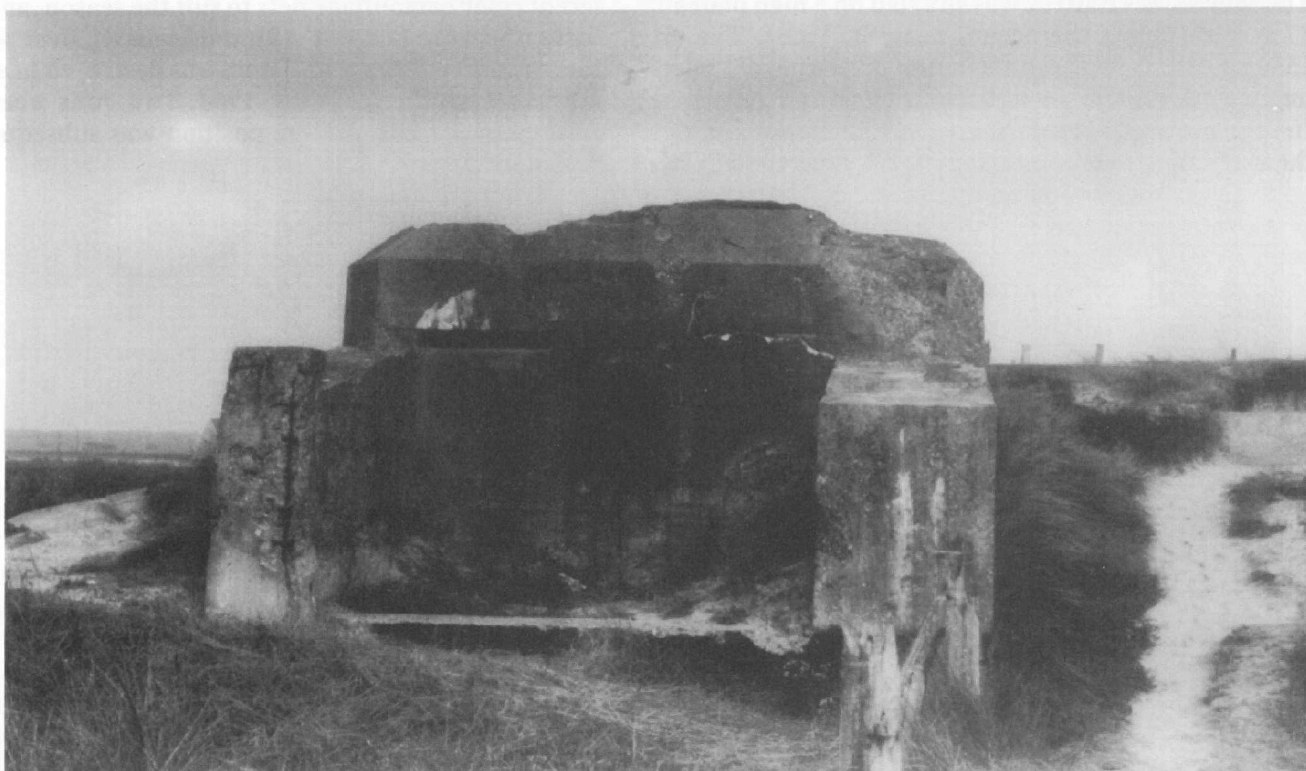
Field-built bunker for the 47mm Pak (t) in the former Resistance Nest 12 as it appears today. The exterior of the bunker shows evidence of numerous hits by enemy artillery, however the ball mount and vision slit are undamaged.
