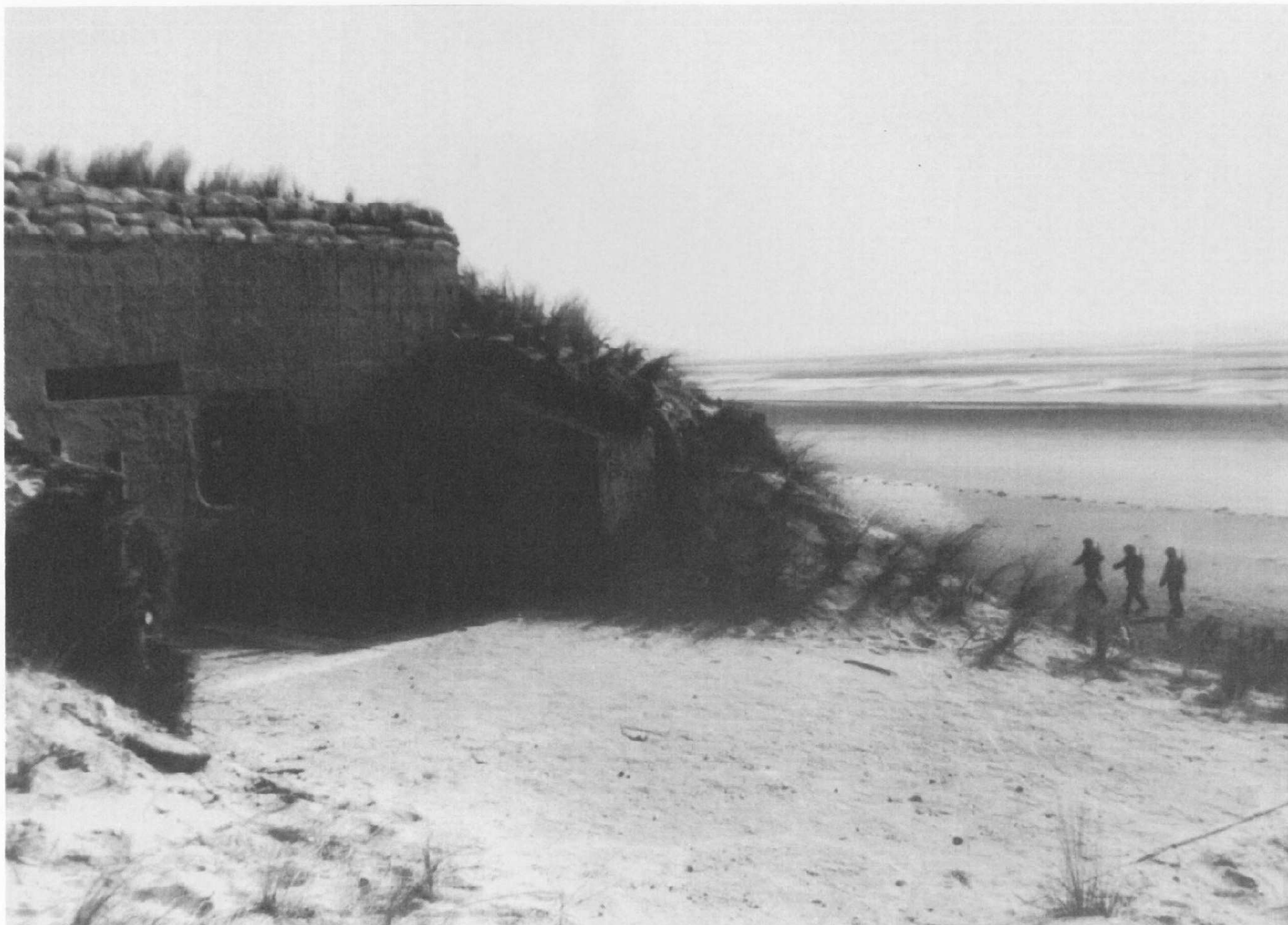
A field-type bunker housing a 47mm Pak (t) anti-tank gun in Resistance Nest 12 near Les Gougins on the Cherbourg Peninsula. The crew of the bunker have reinforced the bunker's roof with sandbags. (BA)
