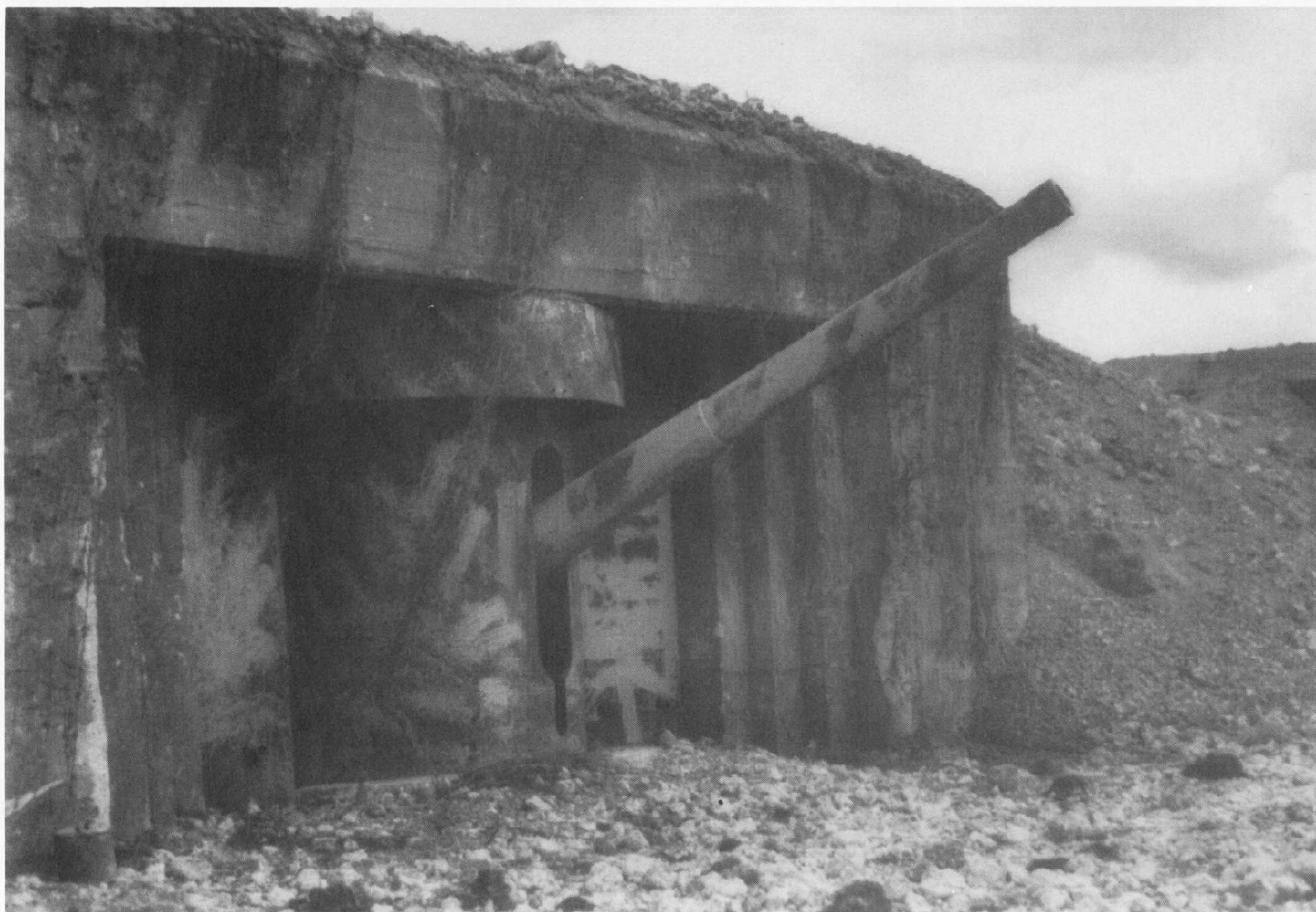
During installation of the 155mm cannon in the bunker, Standard Structure 679, the original gun mount had to be replaced by a revolving mount with embrasure shield. The revolving mount made the gun easier and faster to aim. Below: The same gun bunker on Mont Canisy 50 years later.
